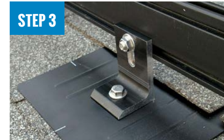
ATTACH L-FOOT TO RAIL
